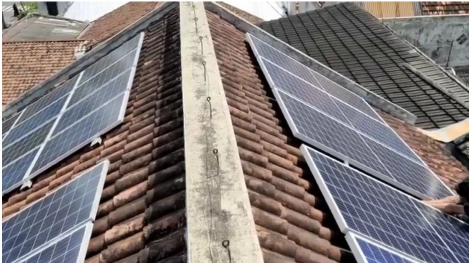
Figure 3. Solar panel Installation Process
