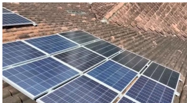
Figure 2. Solar Panel Installation on Community's House Hold (2)
