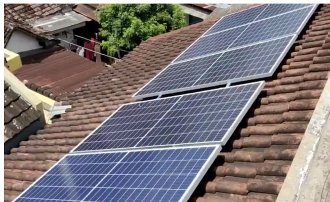
Figure 1. Solar Panel Installation on Community's House Hold
